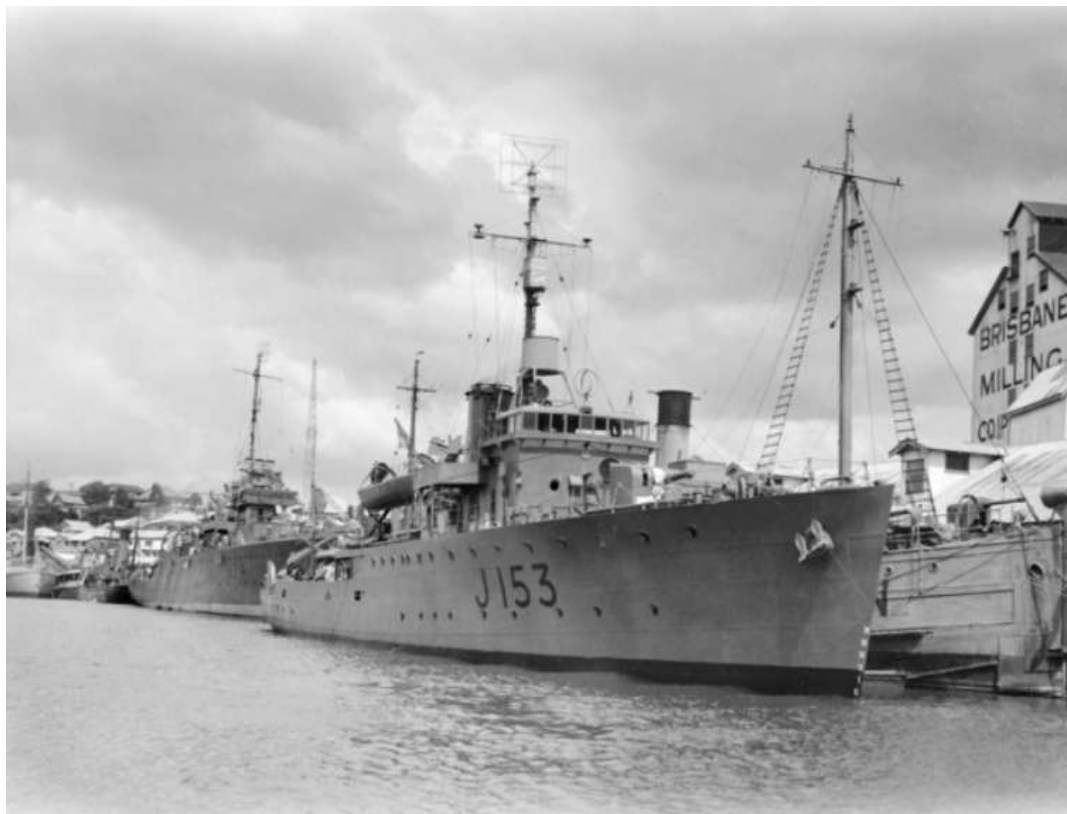
Starboard bow view of Whyalla in Brisbane, Queensland. Behind her is the sloop HMAS Swan. Note a SC radar is fitted to the masthead and a type 272 radar lantern is mounted above and behind the bridge.
