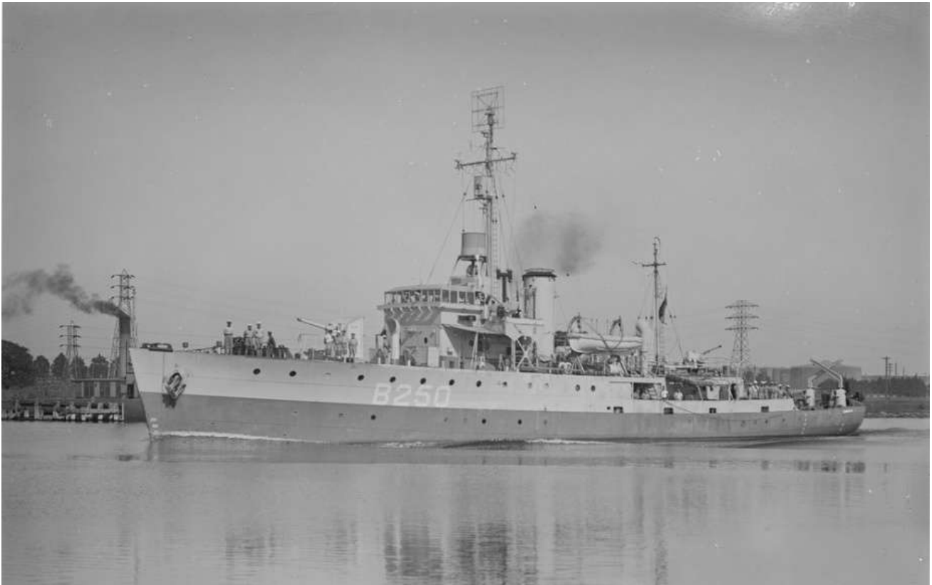
HMAS Tamworth, circa 1945. Note the British Pacific Fleet pennant number preceded by the letter B on her hull. She is also equipped with Type 271 radar, mounted as a 'lantern' at the base of her foremast while at the top of the foremast can be seen her Type 291 radar aerial.
