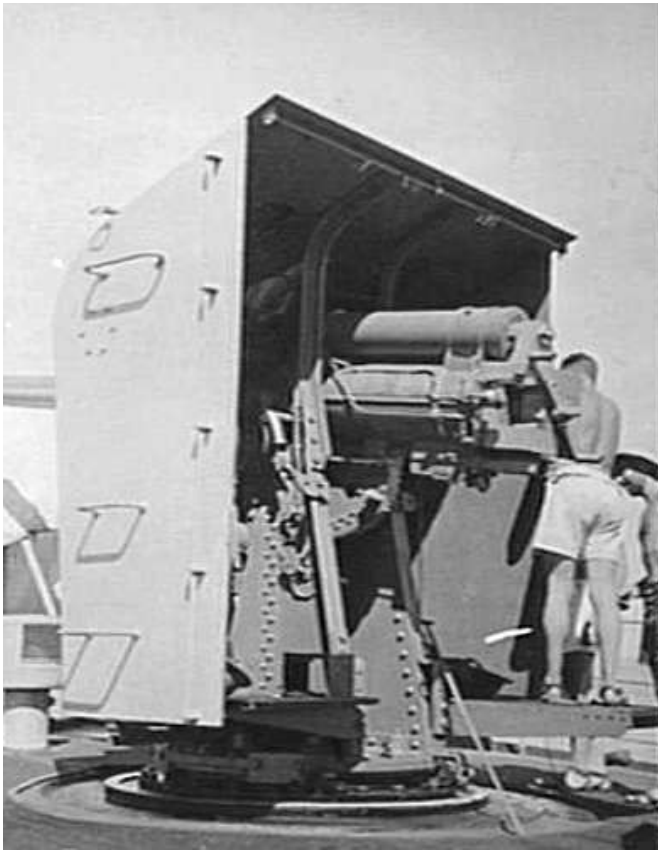
Left: Stawell's 4-inch gun showing breech block and gun shield. Right: To expedite bringing the gun into action, ammunition was kept close by in ready-use lockers fixed on the upper deck. Here Able Seaman J Rapkins can be seen replenishing the locker.
