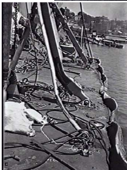
HMAS Mildura lost her motor-boat and had her side bent in a collision with the SS Berwickshire
