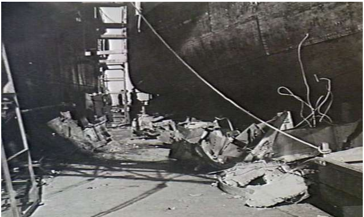
Broken plates on dock floor
