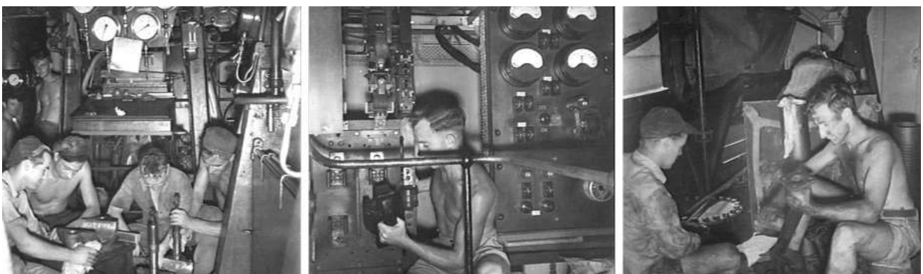
Left: Engine room artificers working on a main engine bearing. (AWM 109338) Centre: An electrician checking gear in the main control room. (AWM 109337) Right: Naval ratings cleaning internal boiler fittings. (AWM 109339)
