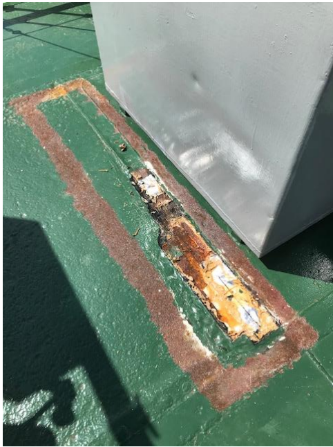
The doubler plate job, a few before, during and after shots.
